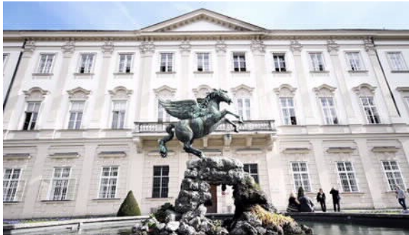
Photo 1: blueSmart manages access control systems at Mirabell Palace, the administrative and government headquarters of Salzburg. Photo: Winkhaus
